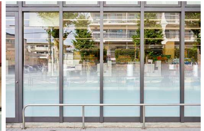
From the outside of the building
